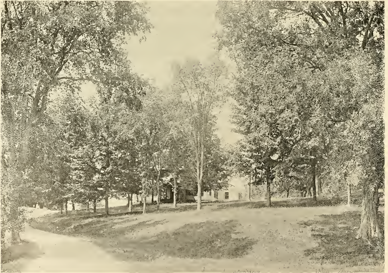
W. P. MACK'S RESIDENCE, LONDONDERRY,—VIEW FROM THE SOUTH.
